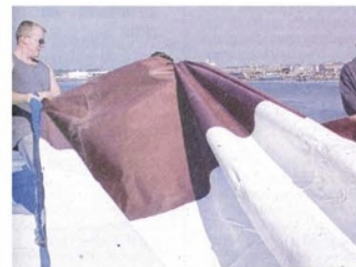
⑥ One at a time, tarps are unrolled and spread over the pile. Each tarp is approx. 60' x 250'.
