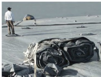
⑤ Vinyl tarps are carried by loaders to the top of the pile. Each roll weighs approx. 500lbs.
