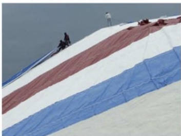
⑦ One at a time, tarps are laid over the surface of the salt pile.
