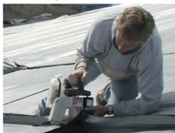
⑪ Adjacent tarps are stitched together with an electric sewing machine like panels in a quilt.
