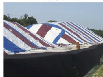
⑫ The final cover is a waterproof skin that snugly encases the unique contours of the salt piles.
