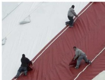
⑧ Weighted bags are tied onto cables that are pre-laminated into the tarp.
