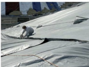
⑩ A seamster climbs up and down the pile along the seams between tarps.
