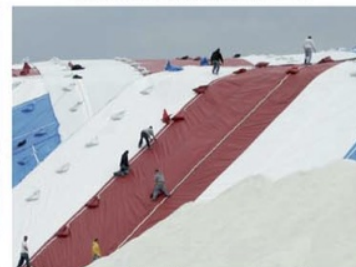
⑨ The weighted bags are placed in an approx. 10' grid that holds down the tarp against uplift.
